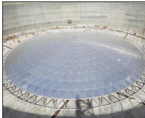
NWC's Faisaliah Concrete Tank, Jeddah, Saudi Arabia (ID 120m x 4 Tanks, 2017)
