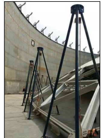
Assembling work, TGSW site, Riyadh
